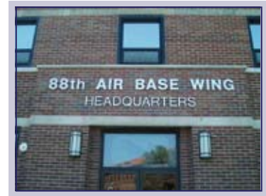
Wright-Patt Air Force Base/Dayton, Ohio-Exterior Wall Sign-cast metal letters with anodized finish.
